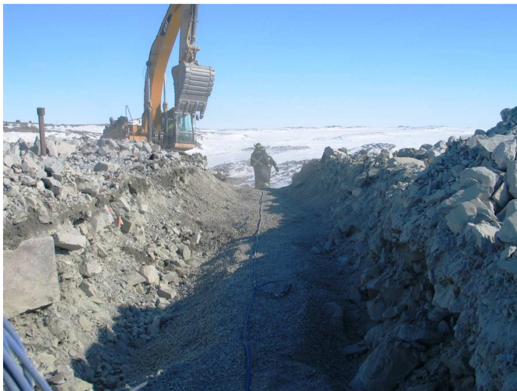
Photo 5: Cable placed across dam at Sta 0+60 US
