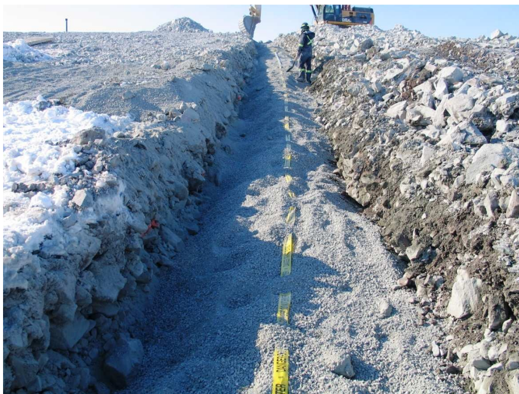
Photo 6: Final lift of crush Sta 0+60 US
